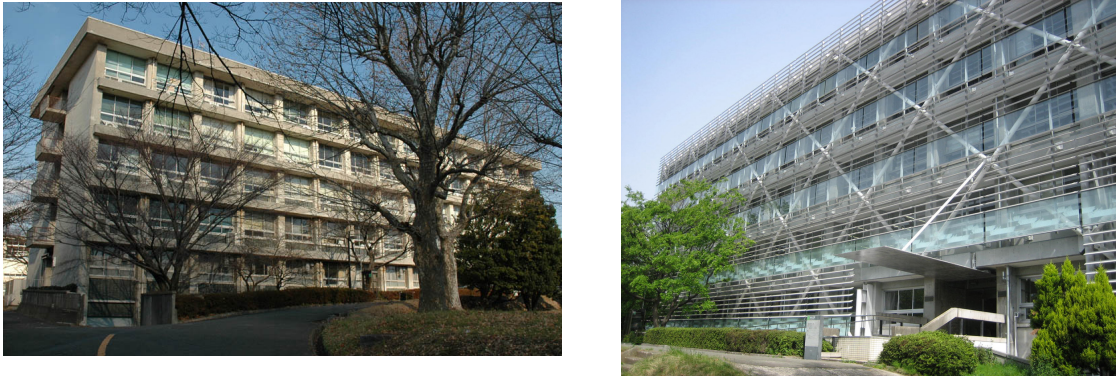
Fig.9 Retrofit of existing RC building with BRBs (before and after).[30]
