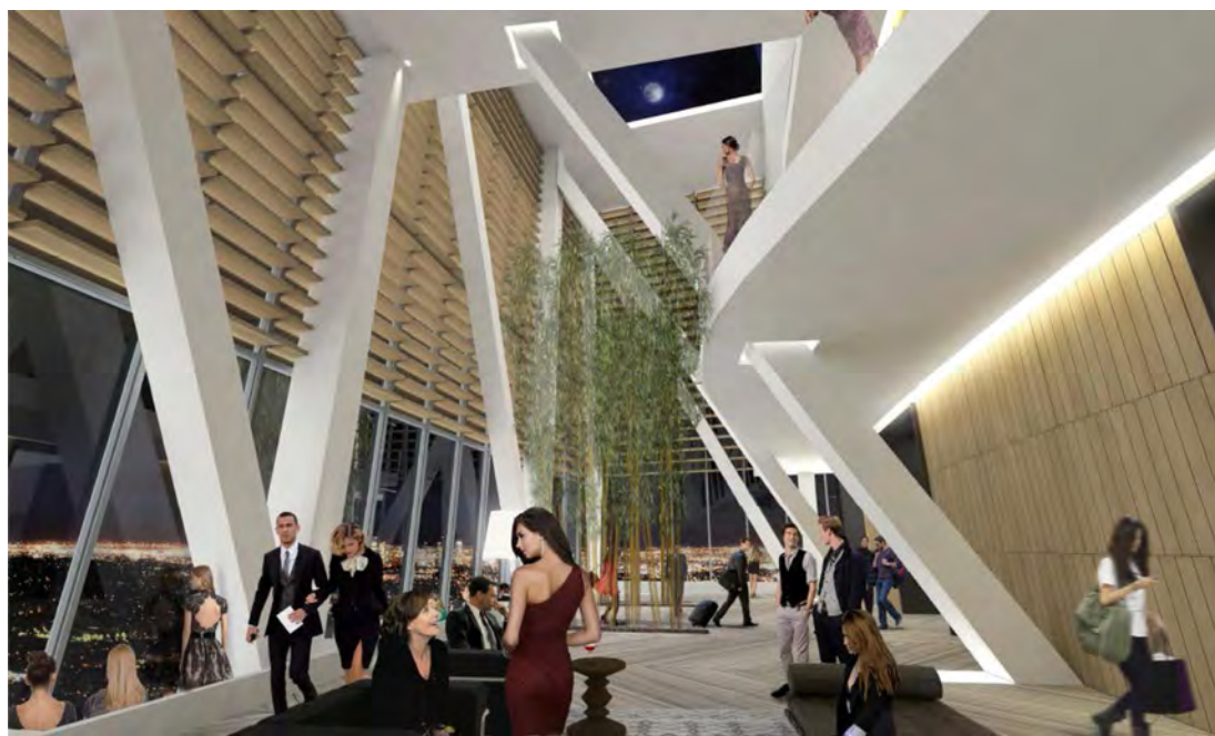
Figure 6. Top outriggers and belt trusses in the Level 70 hotel lobby. Rendering courtesy AC Martin.
