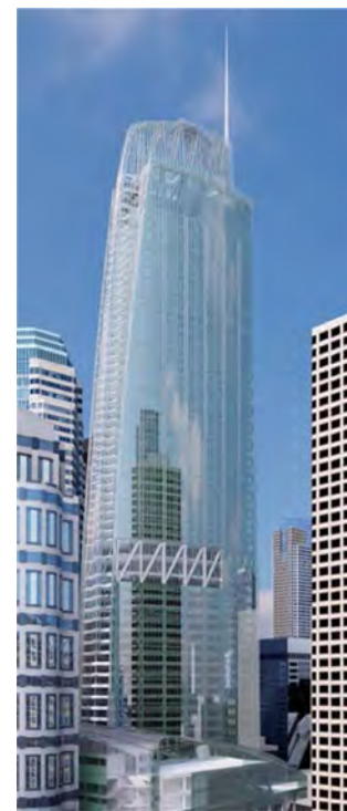
Figure 1. Rendering of the Wilshire Grand tower by architect AC Martin. Note belt trusses, expressed at bottom outrigger level and behind glazing at top outrigger level. Courtesy AC Martin.
