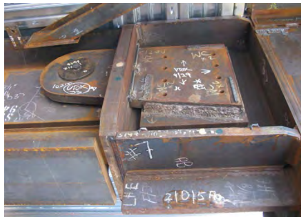
Figure 17. Middle outrigger girder pin at column.
