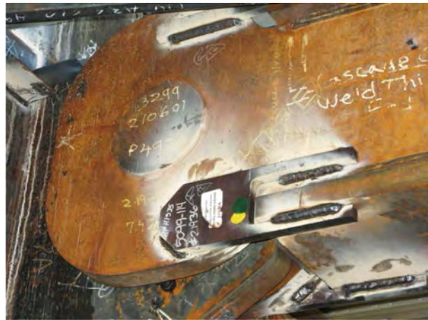
Figure 16. Middle outrigger girder pin at core wall.
